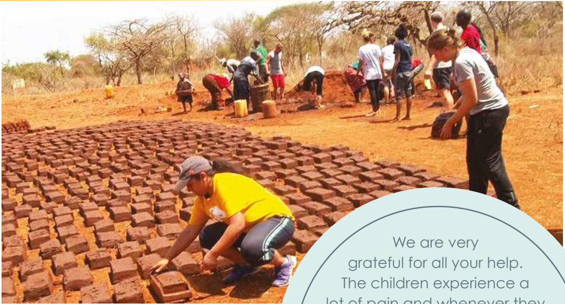
HYC members laying bricks during a brick making exercise
